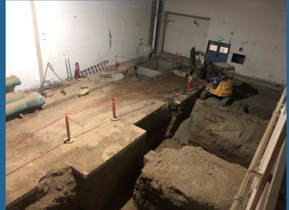
Excavation for underground HVAC in Sector B (room 118)
